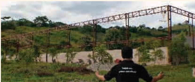
A 5,000-person capacity auditorium, scheduled for completion in May, will serve the Church of God (Seventh Day) in El Salvador.
